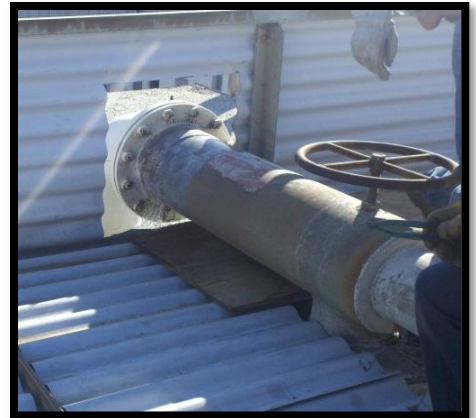
Pipe prepped for repair
