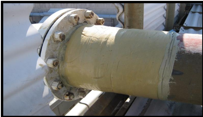
View of Completed Repair
