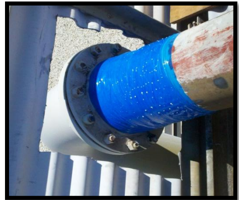
Repair Applied and Curing
